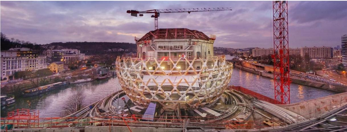
The sail and its mechanisms are in place, the auditorium's glass walls are being finished, tests on the sail are scheduled during December.
