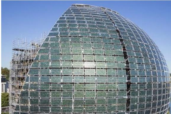
This is how we came to work on the APD, PRO and VISA<sup>4</sup> phases, to support the project players in developing the sail and its mechanisms. The aim being to allow the photovoltaic sail to move around an axis following the sun's azimuth, thereby keeping the sail optimally aimed at the sun. The sail will generate electric power as well as masking the sun shining on the auditorium and acting as a sunshade.
